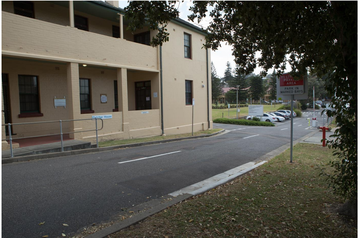
Figure 9.11 Main entrance to Domain. Roadway bitumen and concrete curb repaired after sinking occurred due to early coal shaft that exists under roadway (Wallis Shaft). Source: Charles Hardy, 2014.
