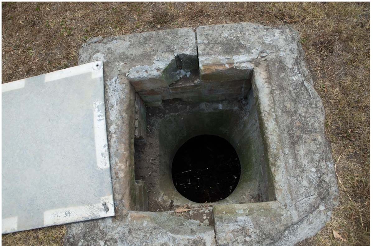
Figure 9.12 Entrance to underground water tank located in front of the workshops at end of main drive. Source: Charles Hardy, 2014.
